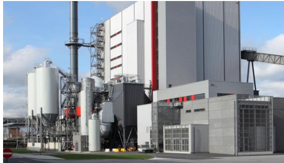
Valmet's CYMIC boiler at Stora Enso Langerbrugge
