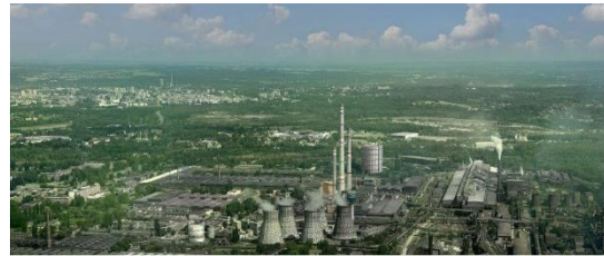
A boiler plant to ArcelorMittal Energy Ostrava s.r.o.
