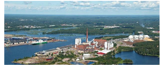
Second commercial installation of Lignoboost™ lignin recovery, Stora Enso
